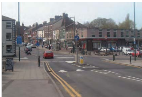
Photo 3.6.3: Mini-roundabout on raised junction
