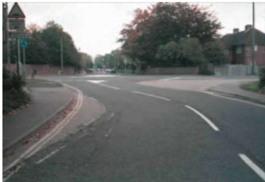
Photo 4.2.9: Mini-roundabout with overrun area
