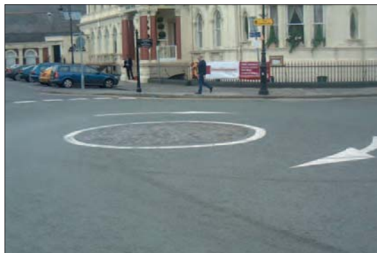
Photo 2.1.6: Non-conforming central marking in setts with white edge marking
