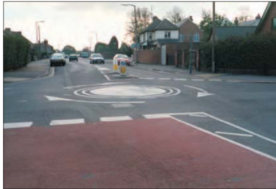
Photo 2.1.3: Non-conforming concentric rings
