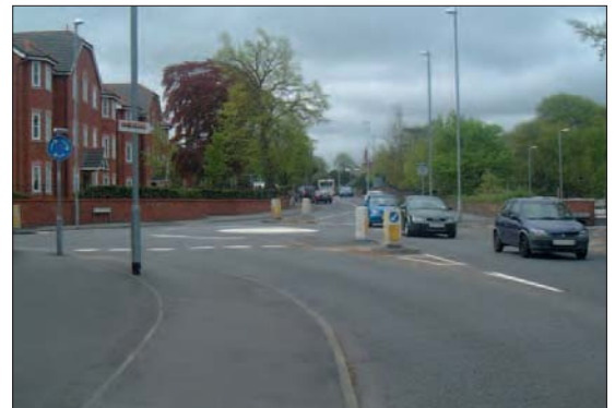
Photo 4.2.6: Approach deflection through alignment and traffic islands
