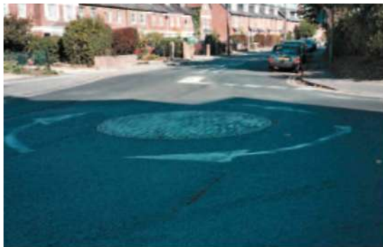
Photo 4.5.2: White paint wearing on blockwork central island
