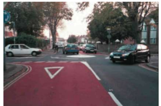
Photo 4.2.10: Mini-roundabout with red anti-skid
