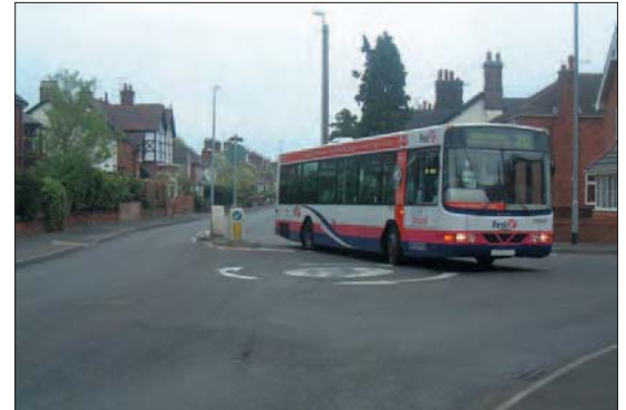
Photo 3.13.1: Bus at mini-roundabout with severe deflection
