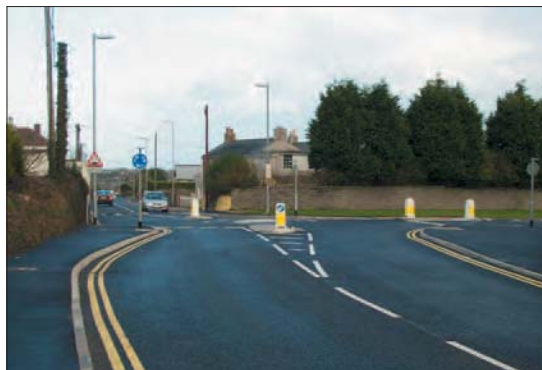
Photo 4.2.4: Deflection through alignment and traffic island
