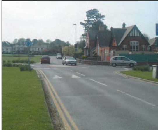
Photo 3.5.1: Site with 'excessive' visibility on raised junction to encourage reduction in approach speeds
