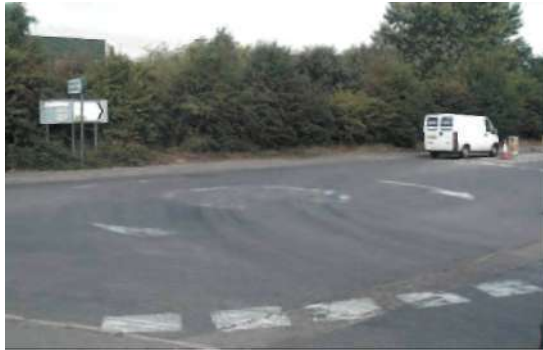
Photo 4.5.1: Poor lining maintenance indicating frequent central island overrunning
