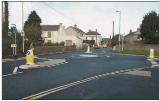
Photo 2.3.2: After view of junction with mini-roundabout
