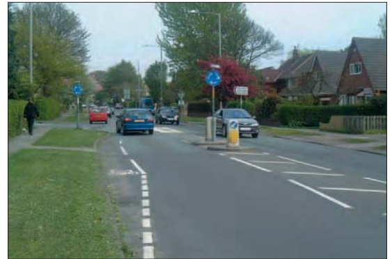
Photo 4.2.5: Approach deflection with kerb alignment and traffic islands
