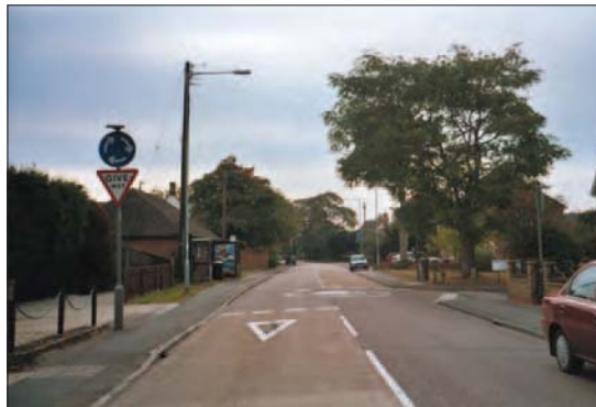
Photo 4.2.3: No deflection on approach or through junction
