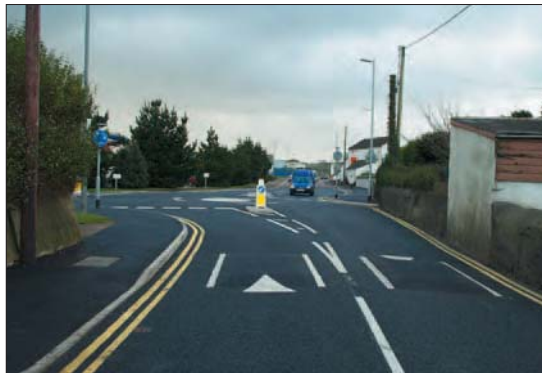
Photo 3.13.4: Traffic calming on approach to mini-roundabout
