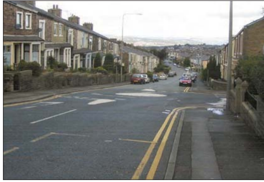
Photo 3.3.1: Constrained site where all vehicles from side road have to overrun central island
